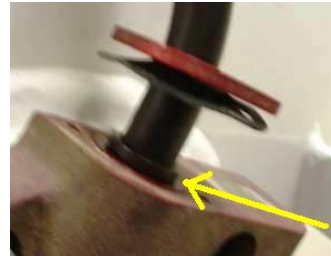
WRONG – LOCKING RING EXPOSED!
