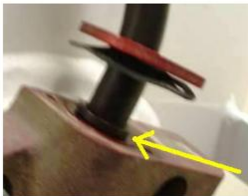
WRONG – LOCKING RING EXPOSED!
